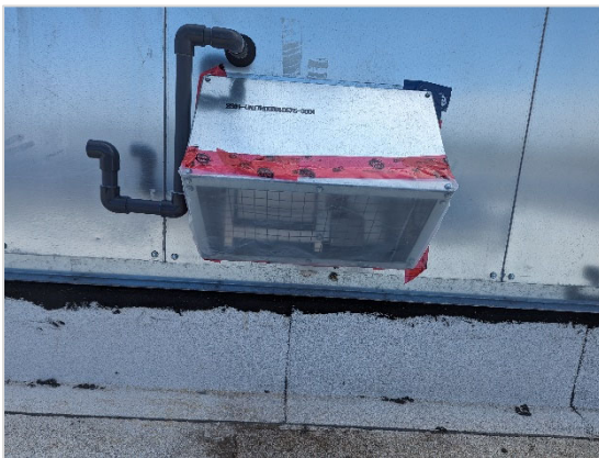
Figure 2: Example of exterior penetration sealing at make-up air unit
