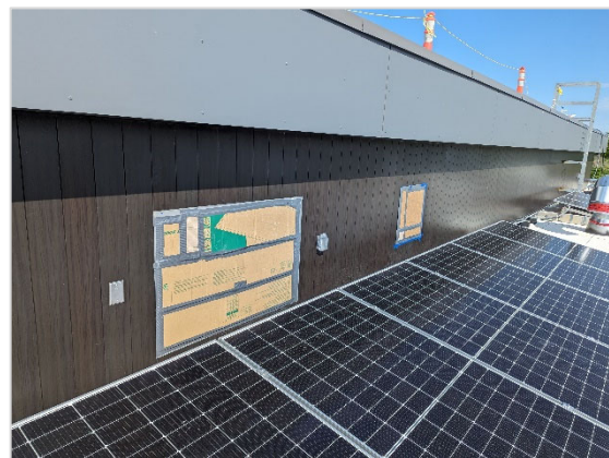
Figure 3: Example of exterior penetration sealing at exhaust ducts
